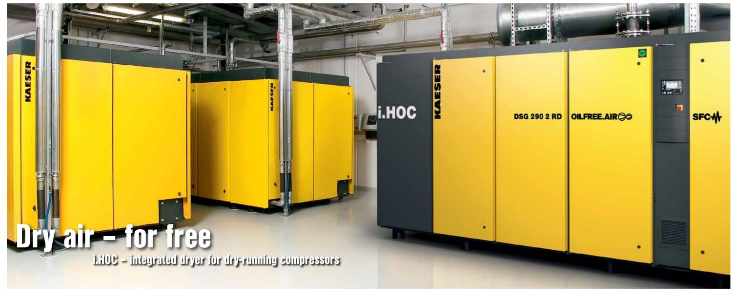
Innovative, intelligent, integrated - the new i.HOC compressed air dryer as an integrated component of a DSG series dry-running rotary screw compressor.
